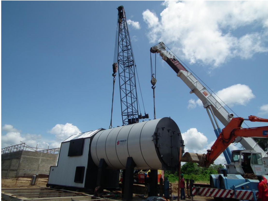
Caption: Installation of furnace and boiler in Apoera
